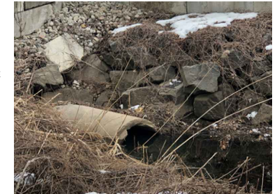
EXISTING CULVERT DOWNSTREAM RIP-RAP
