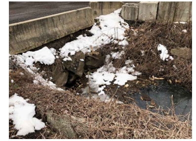
EXISTING CULVERT UPSTREAM RIP-RAP
